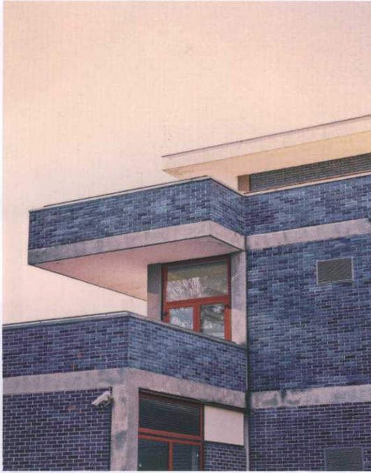
↑ THE CENTRO STUDI ED ESPERIENZE OLIVETTI IN IVREA, DESIGNED IN 1951-55 BY EDUARDO VITTORIA TO HOUSE TRAINING FACILITIES FOR OLIVETTI'S DESIGNERS. SEE PAGE 152
